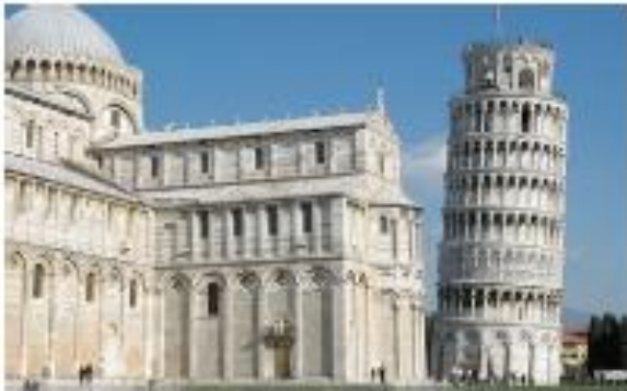
Leaning Tower of Pisa
